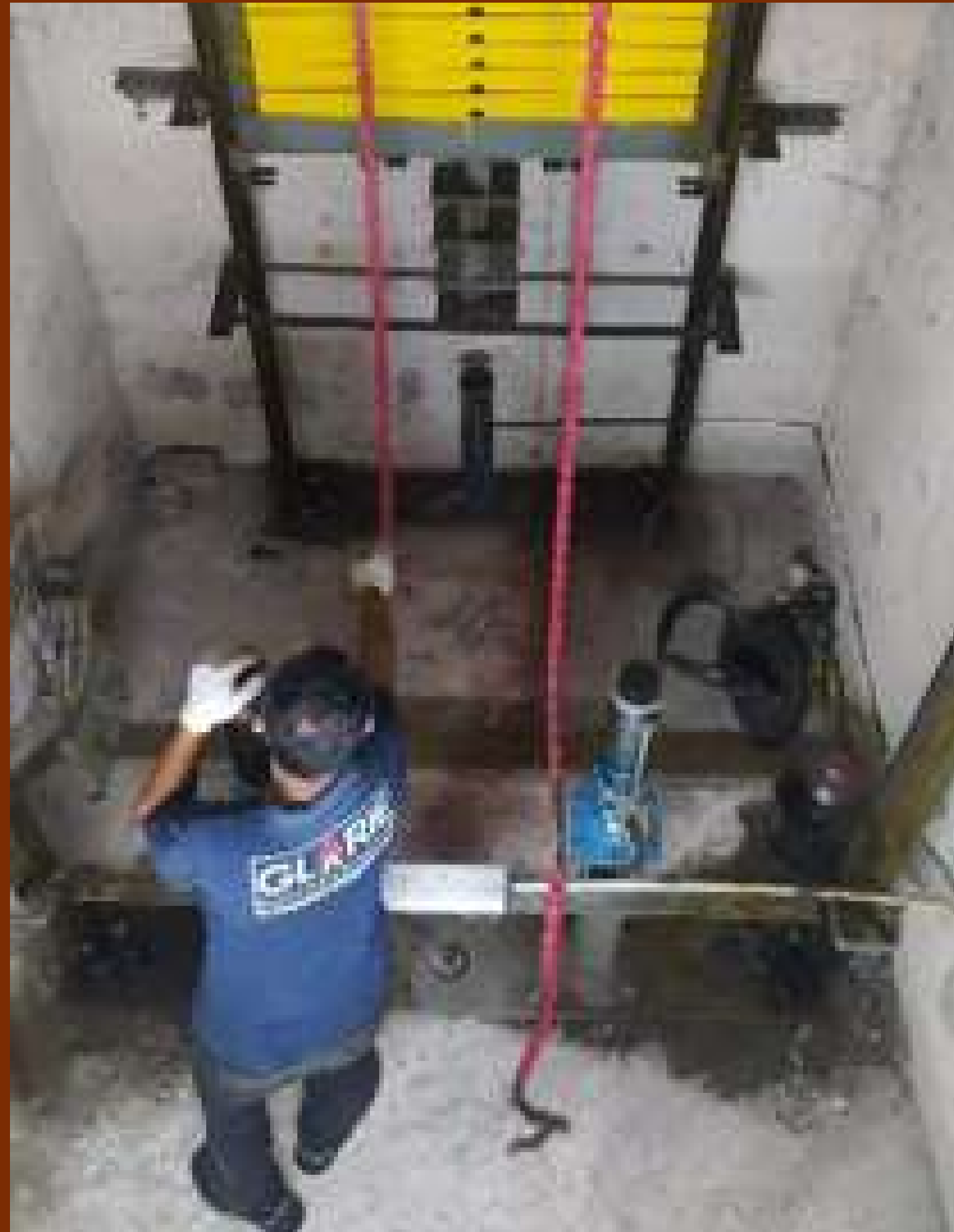
Penggantian Compasating Chain Lift Service Topaz 2
